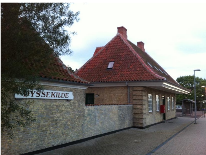
Dyssekilde stationsbygning – p.t. under forbilledlig restaurering
